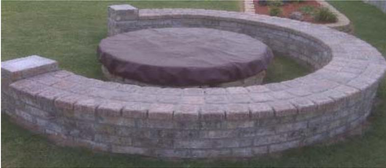
Step 19 → I found some gothic bull nose capping stones for the ends of the seating area and so I added one more row of bricks, set off just a bit so that they would match up with the 13" stones. The project is finally complete after cleaning the brick and sealing it. It was windy so not all the flames are present as they should be in this picture.
