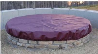
Step 17 → The seating area was bricked. This was my first taste of brick laying and while I would suggest to a novice to start out with a straight wall for the first time, I eventually got the hang of the curve and it went along pretty quickly. I am pleased with how it turned out.
