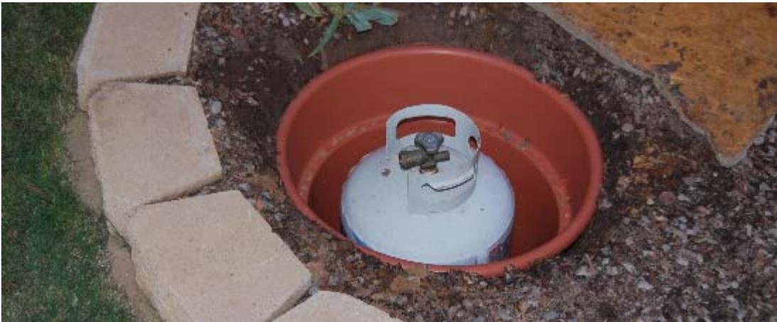
Step 7 → A form (plastic border for flowerbeds) was put around the inner circle of the fire pit to hold in the concrete. 4 bags of Quickrete were used, it dried over night and then the form was broken free.
